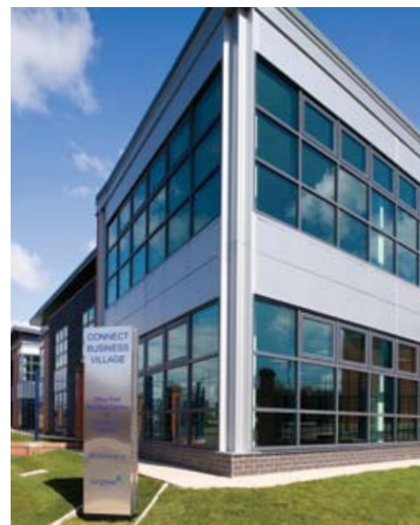
Self contained offices
