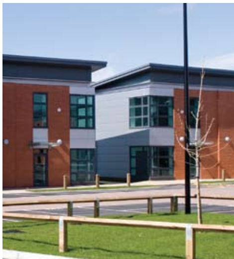
Self contained offices
